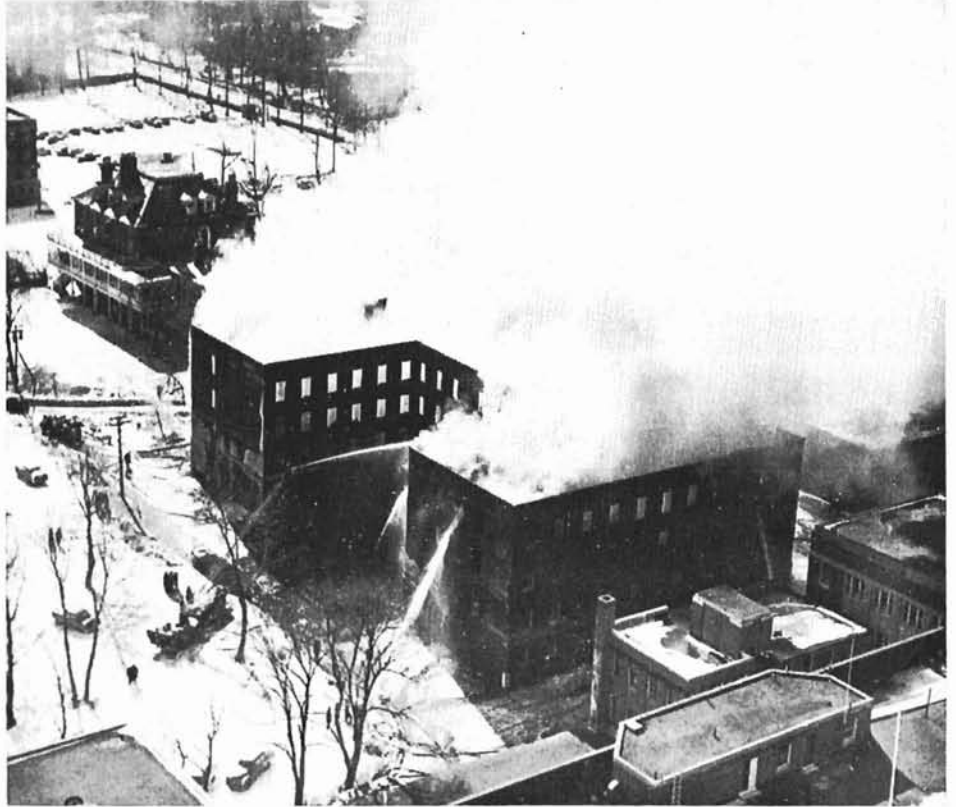
An alert fire sentry (AB Roy Turner) and the discipline of the 127 men in the building won credit for the absence of loss of life when fire which broke out at 3 a.m. destroyed the chief and petty officers' living block at Stadacona on February 27. Residents had to flee so quickly—some of them by sliding down ropes from the third floor—that most of them lost clothing and personal effects. Halifax and naval fire departments kept the flames from spreading to nearby buildings. (HS-22846)
