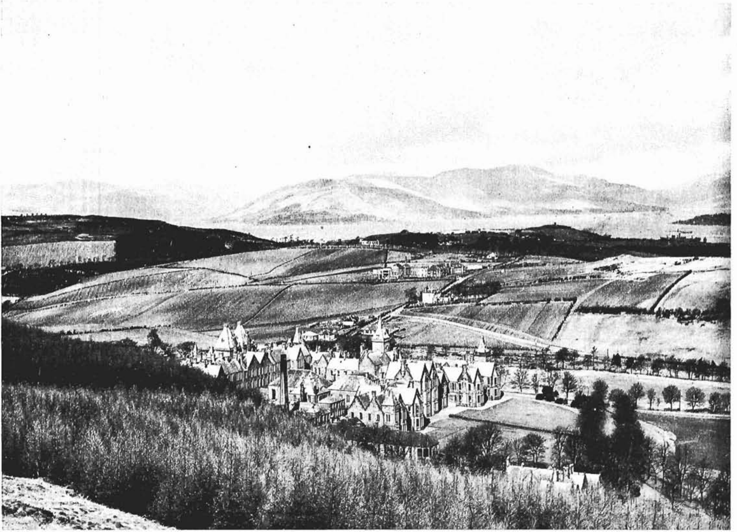
This cluster of buildings, nestling in a valley near Greenock, Scotland, was commissioned during the Second World War as a ship of the Royal Canadian Navy—HMCS Niobe. Although the scene may bring to mind King Arthur's "many-towered Camelot", the establishment was manned by hard-working sailors and wrens, rather than knights in shining armour. (WD-832)
